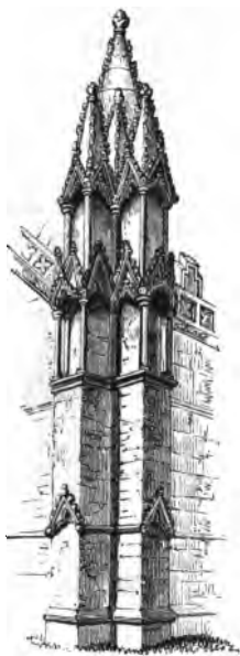
147. Gadsby, Leicestershire, c. 1350. Corner buttress with canopies and pinnacle.
